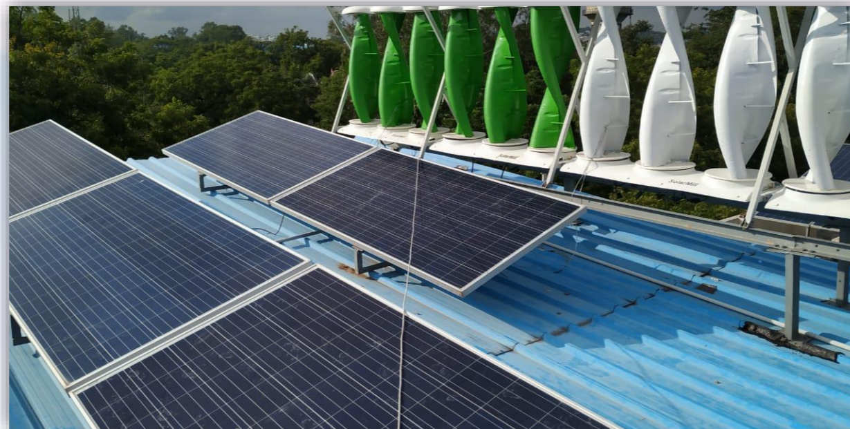
Solar-Wind Hybrid Plant on ESTC
